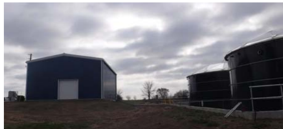
Figure 1. Photograph of the Missouri City Landfill 250,000-gallon storage tanks and the water treatment plant building.
