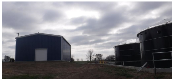
Figure 1. Photograph of the Missouri City Landfill 250,000-gallon storage tanks and the water treatment plant building.
